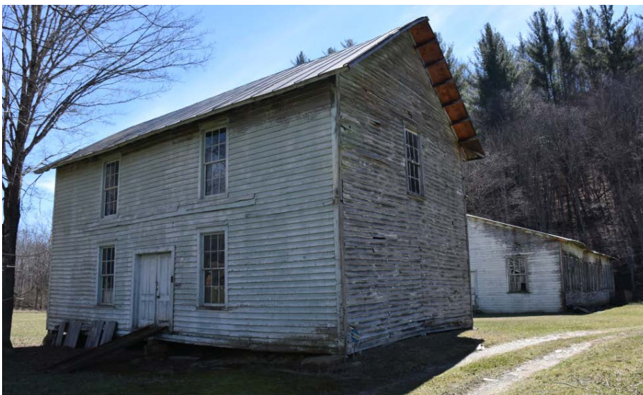
Company Store, northwest oblique
