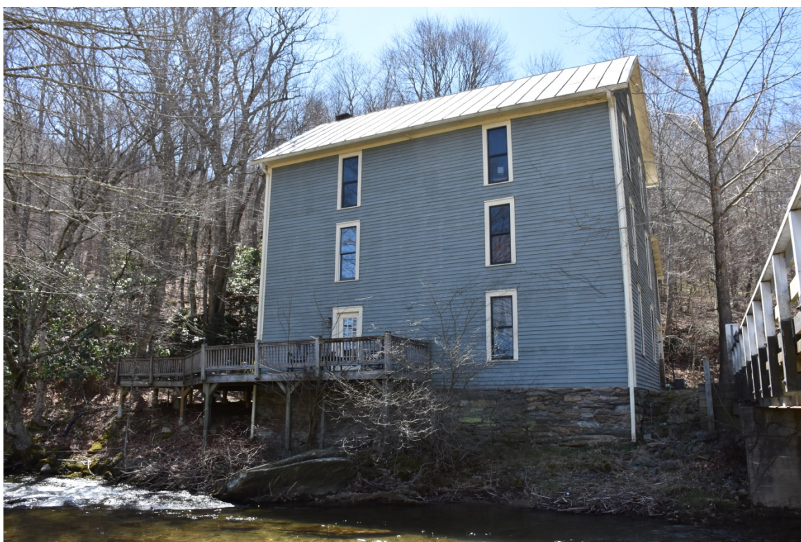
Helton Roller Mill, north elevation
